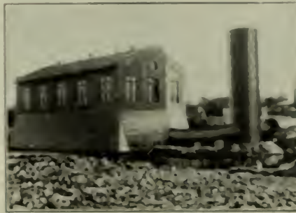
FIG. 2. EXTERIOR OF POWER HOUSE
